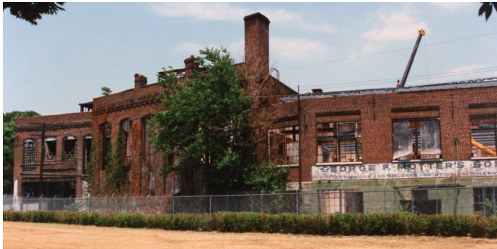
West Princess Street view, formerly G. Motter and Sons
